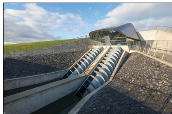
Figure 1.2: The fish-friendly jack screw pumps at De Heining pumping station. The two jack screw pumps form a connection from the storage basin and the polder to the Wadden Sea. (Source: https://www.rijkswaterstaat.nl/water/waterbeheer/wat-erkwaliteit/maatregelen-waterkwaliteit/ruim-baan-voor-vis/vispassage-de-heining#&gid=1&pid=2 )
