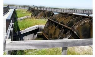
Figure 3 Paddlewheels on the east side of the oyster trench provide waterflow (L. Sanders, 2021).
