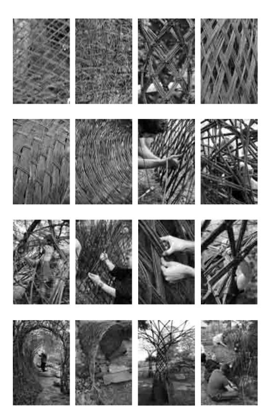
the students started weaving the dome from the centre. As a result, the form emerged of its own accord on the basis of the weaving method. The structure is a 'randomly' woven surface. Adding tension to this structure results in a sturdy rounded shape because the curved wicker branches press inwards. Weaving in a controlled manner results in a geometric shape.
