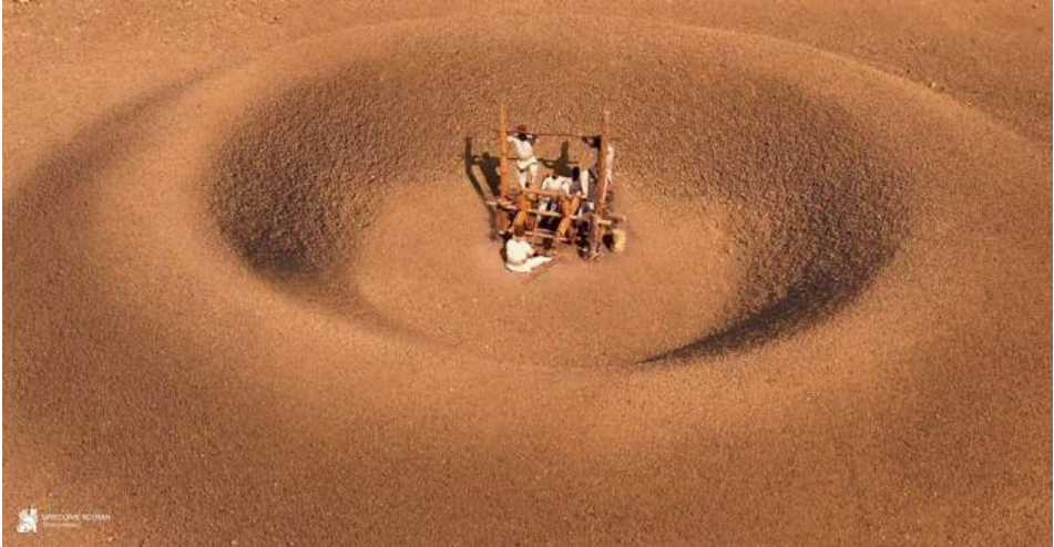
Type of underground irrigation canal between an aquifer on the piedmont to a garden on an arid plain. This system is best known from Iran.
