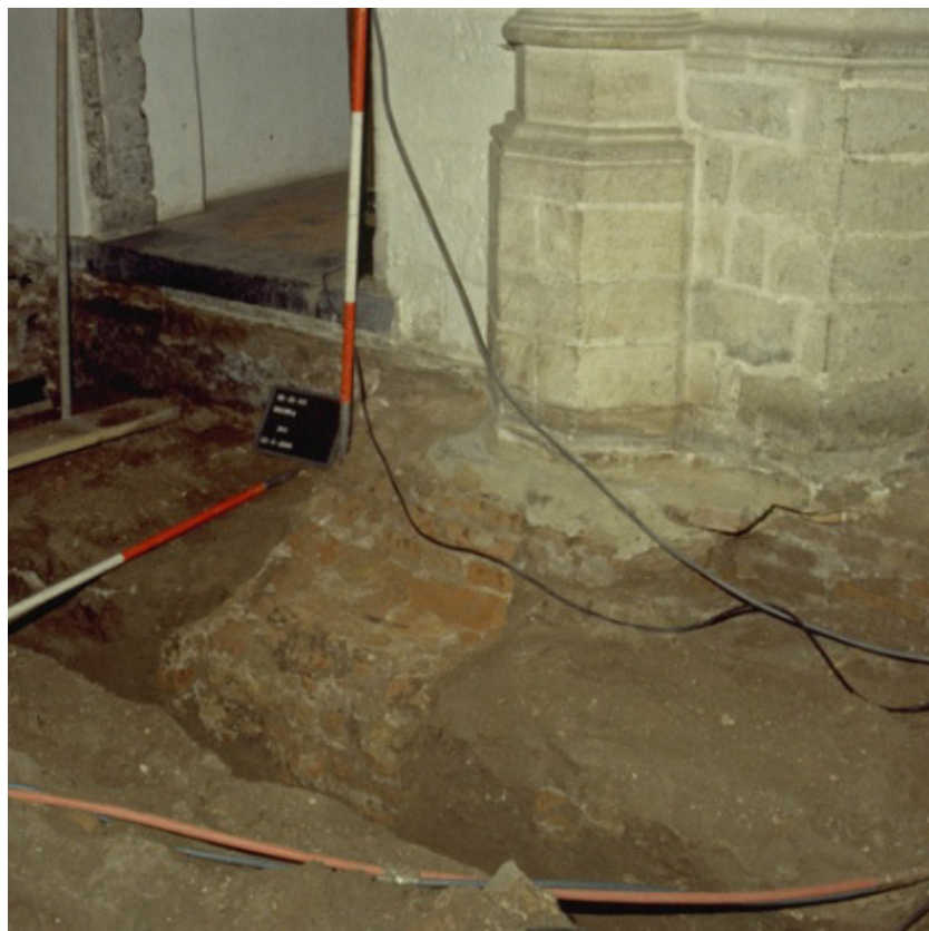
A characteristic of the underground structure is that the foundations run outwards and a different material, brick.
