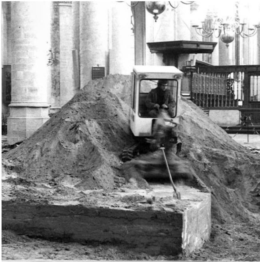
This is during a renovation where the floor of the ship is open. An existing basement is also visible here.
