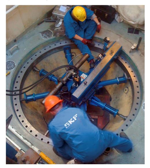
Figure 5-21: Flange facing equipment (SKF, 2013)
