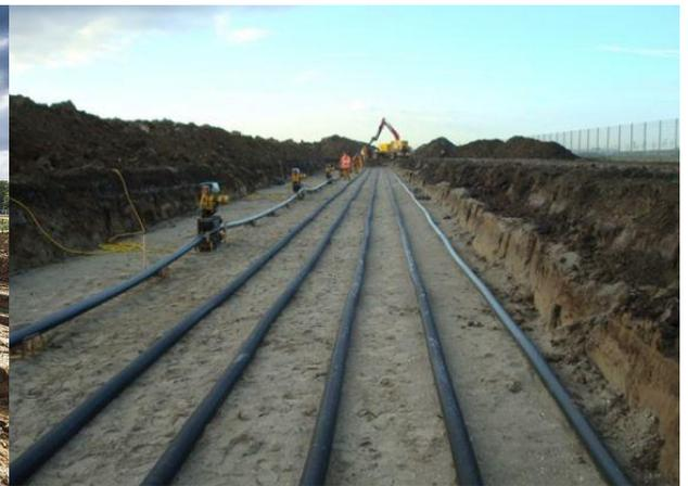
Figure 2-2 Right of way of a 150 kV conventional connection [54]
