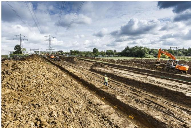
Figure 2-3 Right of way of a 380 kV conventional connection [55]
