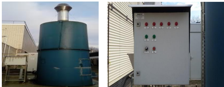
Figure 18 Gas flare & control panel
