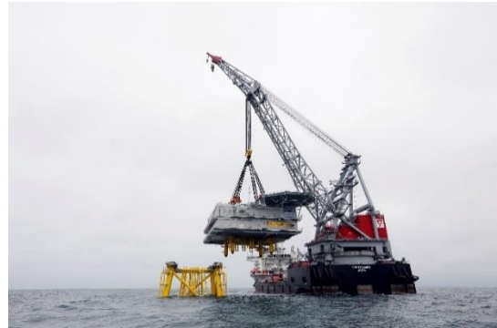
Figure 6 Topside lifting by crane
