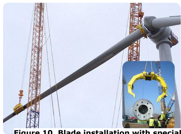
Figure 10, Blade installation with special clamp and two hoists
