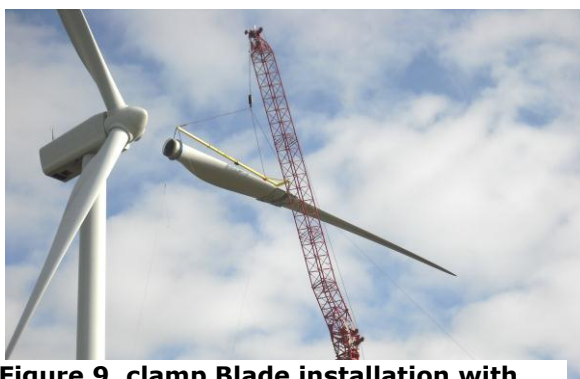
Figure 9, clamp Blade installation with special clamp and one hoist
