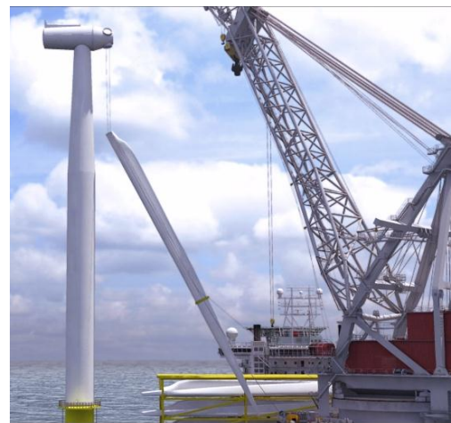
Figure 12, Blade pull in concept
