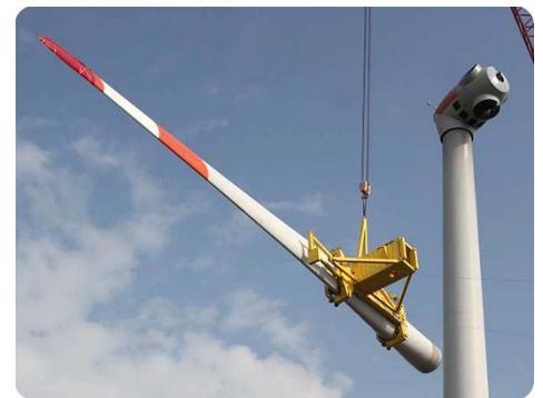
Figure 5, One connection, horizontal blade installation
