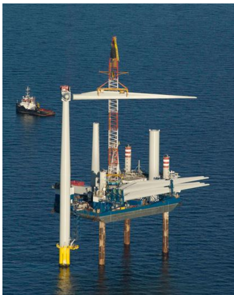
Figure 7, Jack-up blade installation with special clamp
