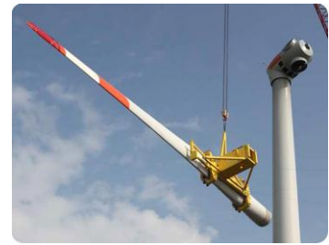
Figure 1, Single Blade installation
