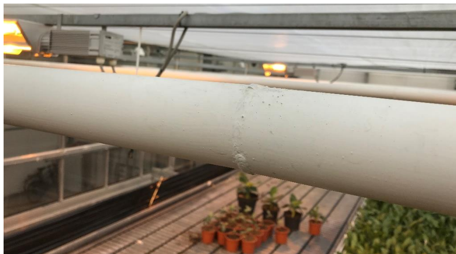
Figure 2 Kink in heat pipes due to welding
