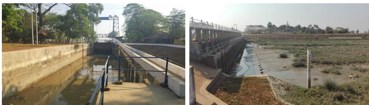
Figure 4: Tawa lock gate and sluice gate in the dry season
