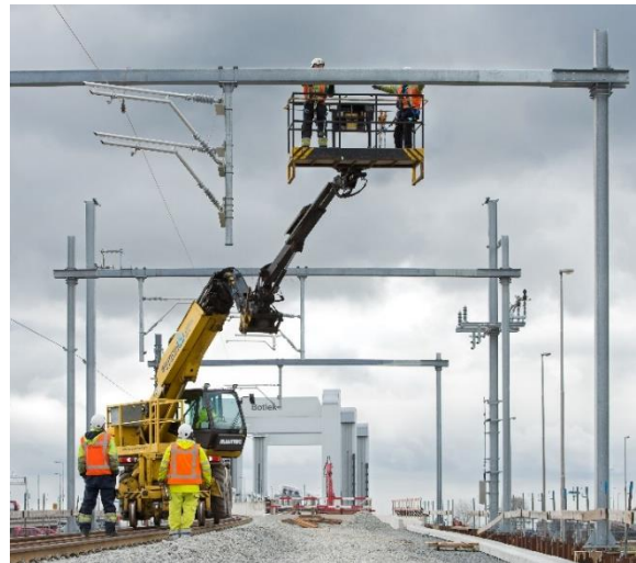
Figure 1. Employees on a KROL working on catenary system (Strukton Rail, 2019)
