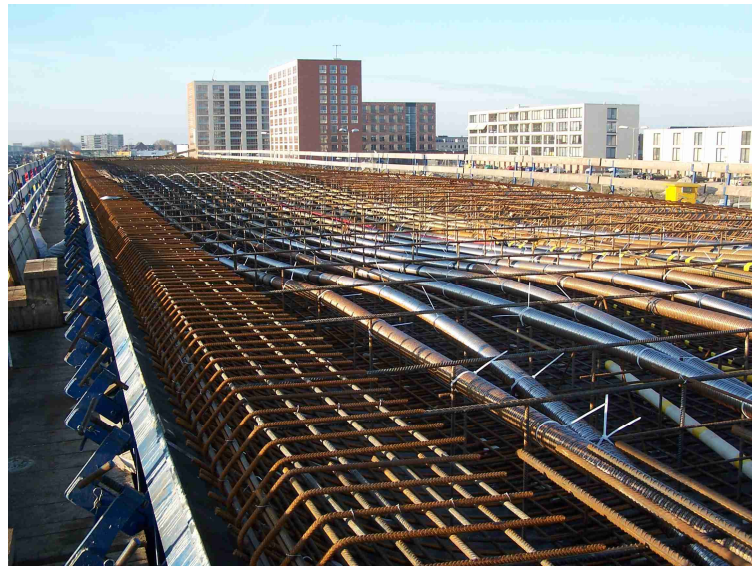
Figure 5.3 Post tensioned cast in place*
