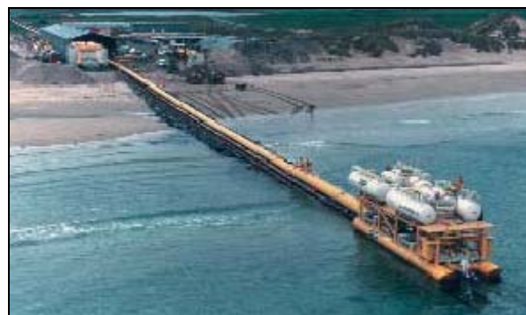
Figure 2.2.3 Controlled Tow method
