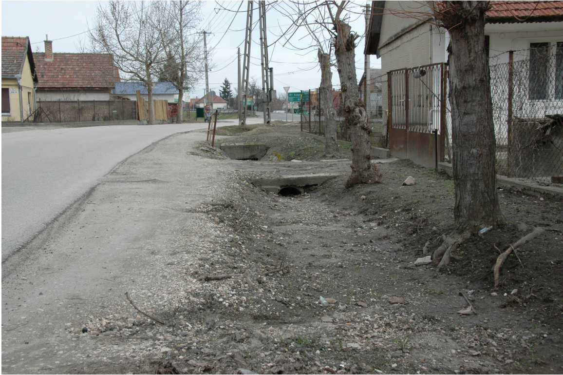
Picture 7: RWD system in state of neglect
