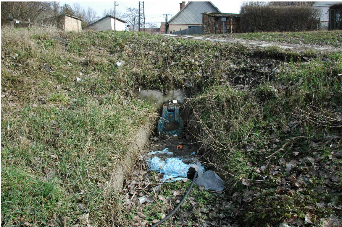
Picture 8: outlet 5 (see map 3) RWD system, silted up with sand and trash
