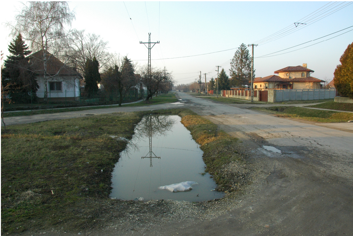
Picture 6: filled up RWD system almost causing inundation of the roads, Dömsöd
