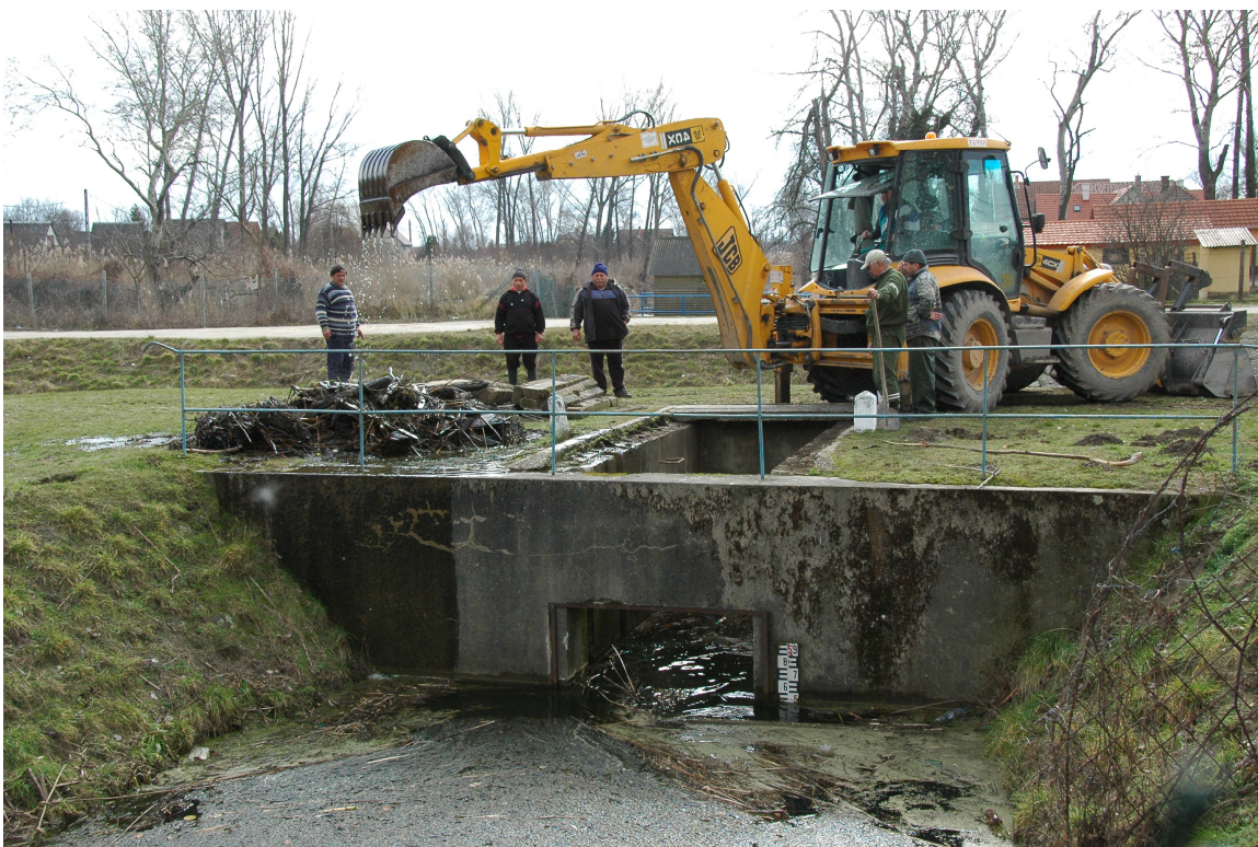
Picture 9: cleaning the jammed siphon under the irrigation canal, March 2010
