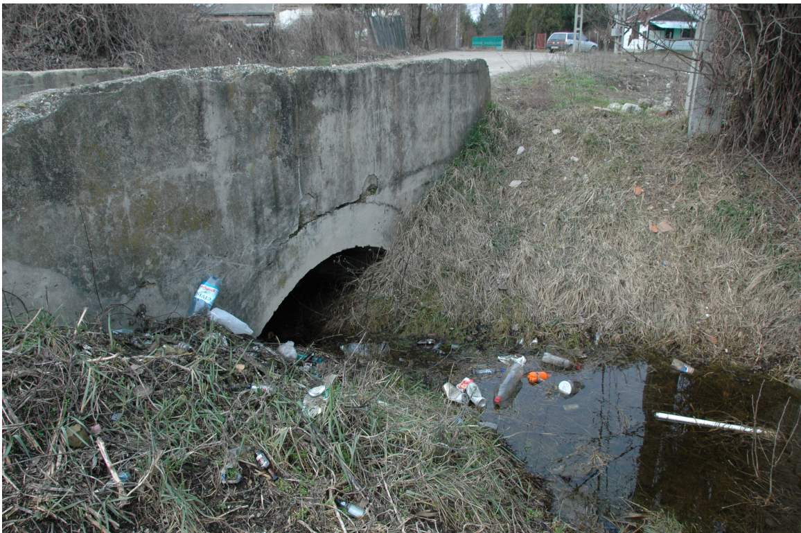
Picture 18: bridge over the Tókert canal what might need re-dimensioning.
