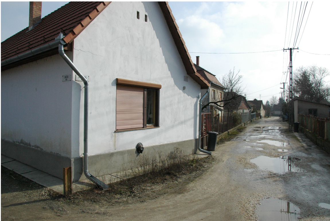
Picture 22: rainwater from roofs in present situation; discharging on the road
