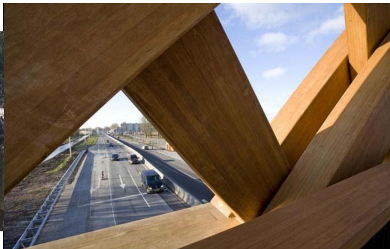
Figure 4.6 Sneek bridge made of finger-jointed and laminated Accoya.
