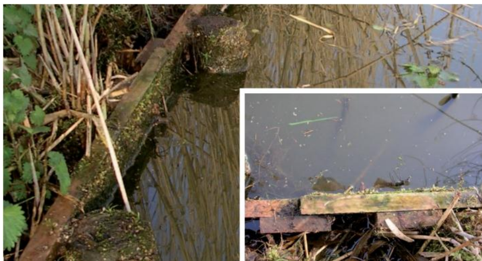
Figure 4.7 Accoya post to board as shore protection construction waterway in Flevoland.
