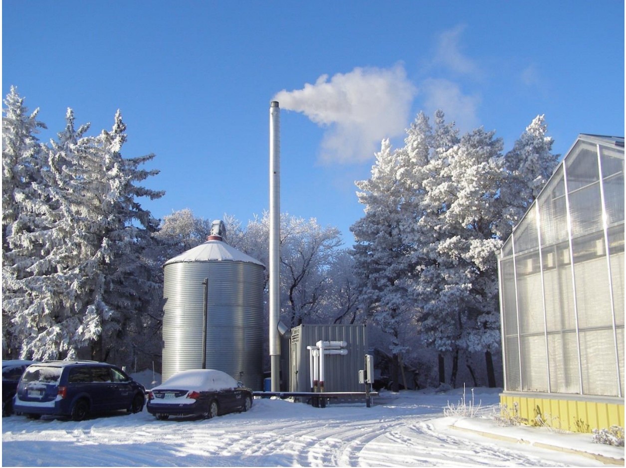
Figure 3.7: The containerized wood-fired boiler plus storage silo at the ADC in Indian Head
