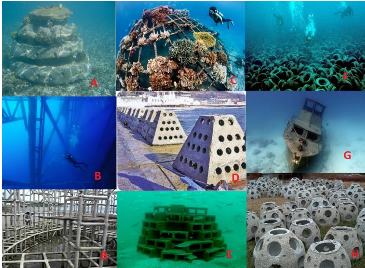
Types of artificial reef structures found: A= Layered Cake, B= Metal structures (diverse), C= Biorock, D= Concrete pyramids, E= Concrete blocks, F= Tires, G= Wreck, H= Reef balls
