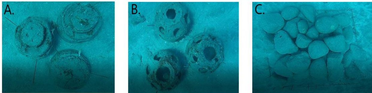
Figure 2 : Artificial reef types used in the AROSSTA project: A.= layered cakes, B.= reef balls ,and C.= Rock reef
