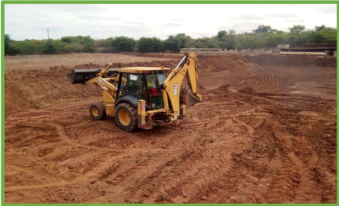
Picture 13: Construction of a 30m X 40m pond
