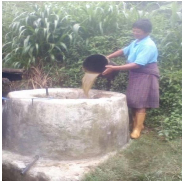
Figure 5: Feeding the digester with dung and Biogas
