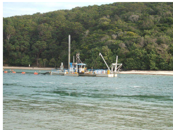
Figure 8: Dredging at Tallebudgera Creek (Source: Neumanncontractors, 2015)
