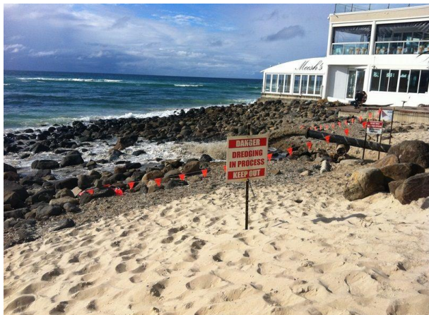
Figure 7: Sand is moved from Tallebudgera Creek onto Burleigh Beach (Source: Neumanncontractors, 2015)
