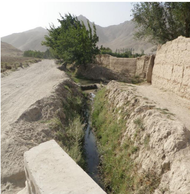
Figure29 poorly maintained Afghani Canal
