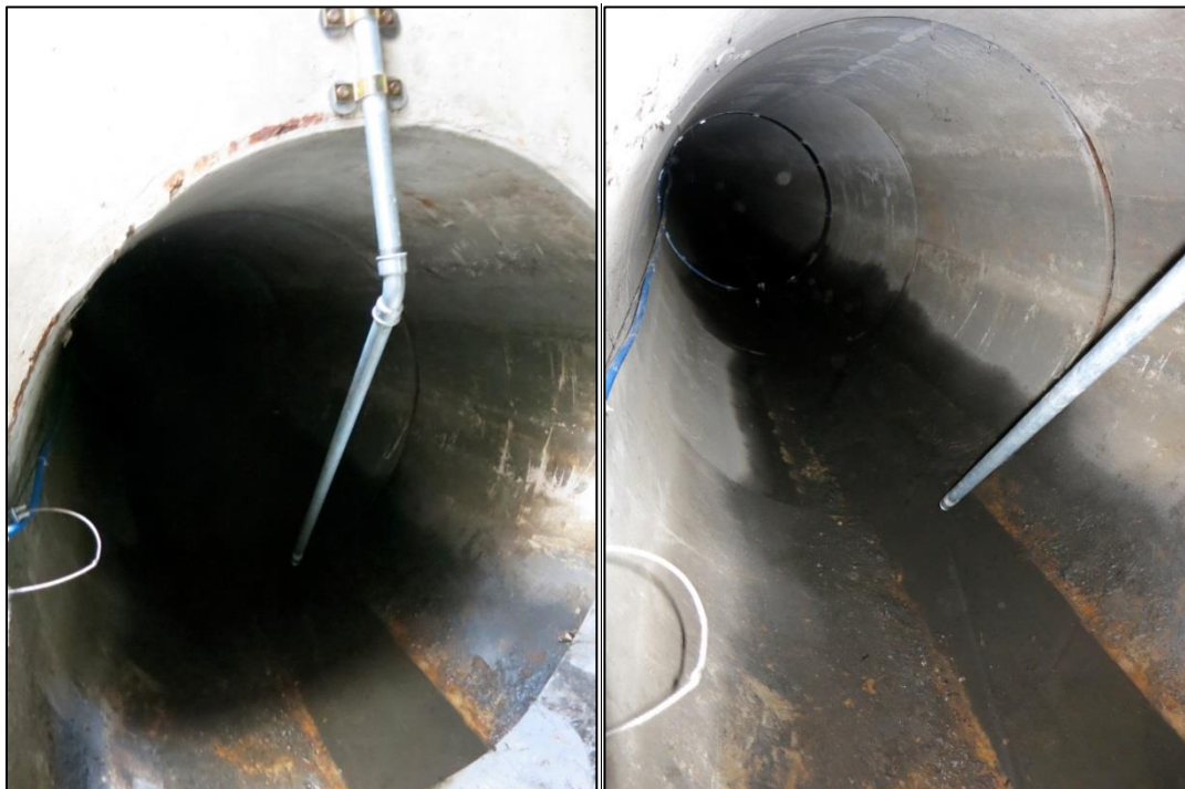
Figure 28: Steel pipe that leads sampler tube into the sewer into the direction of flow.
