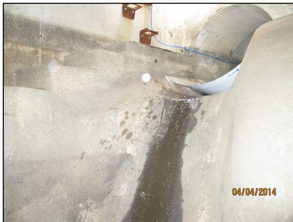
Figure 27: Installed steel plate, seen from downstream.
