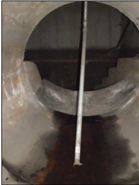
Figure 29: Blockage of the sampling tube.
