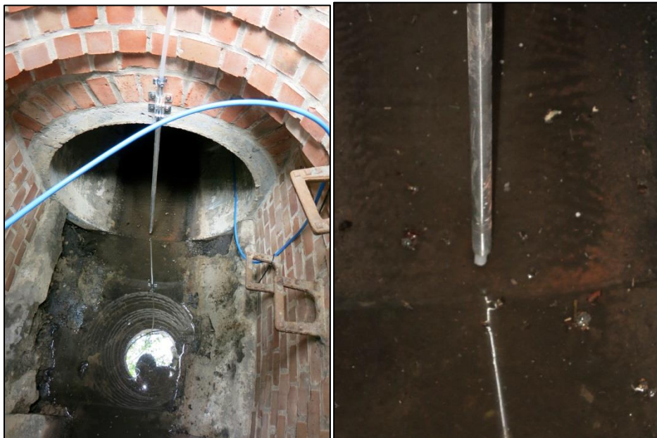
Figure 16: Installation of the steel pipe that leads the sampling tube downwards.
