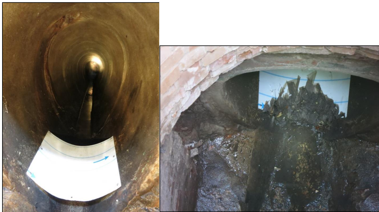
Figure 22: Lower part of steel plate lifted from bottom and effects, blockage still occurred.
