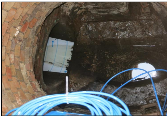
Figure 21: Steel plate causing permanent backwater.
