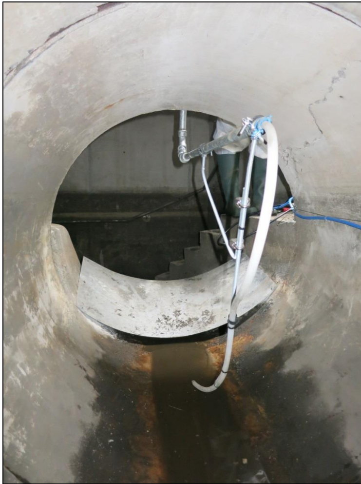
Figure 30: Situation after modifications, steel plate is lifted and sampling tube pointing in downstream direction.
