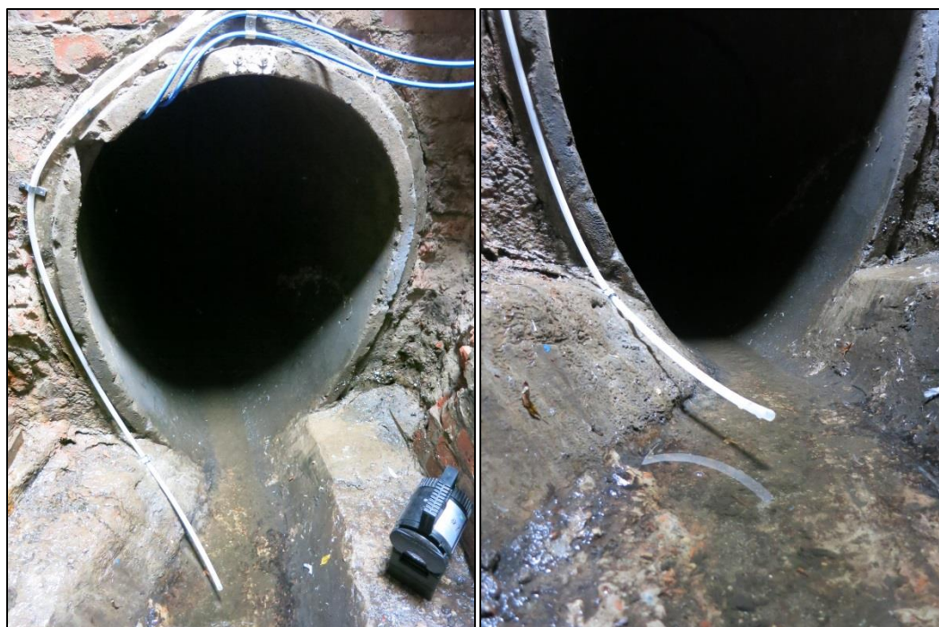
Figure 23: Improved installation, preventing the trapping of litter.
