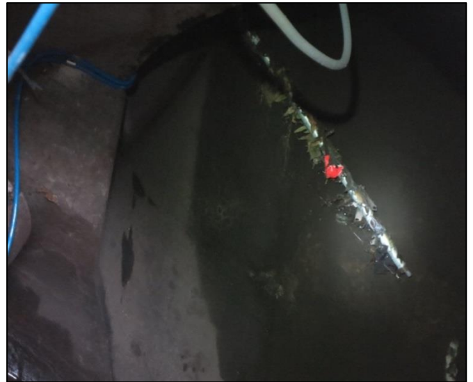
Figure 25: Litter trapped on steel pipe, end is still clean.
