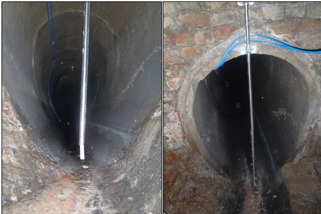
Figure 19: Initial installation of steel pipe and sampling tube.
