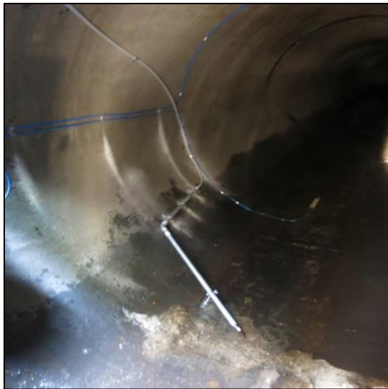
Figure 24: Sampler tube and steel pipe after installation.
