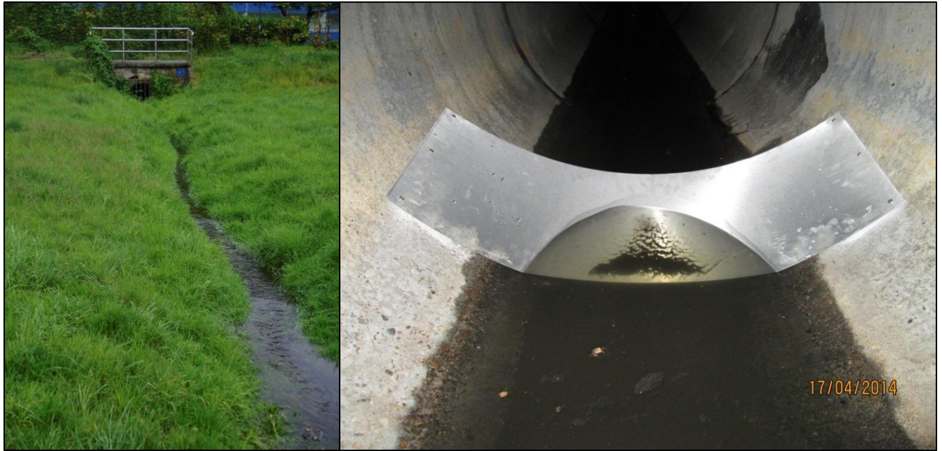
Figure 17: Steel plate fixed to channel bottom, open channel not cleaned.
