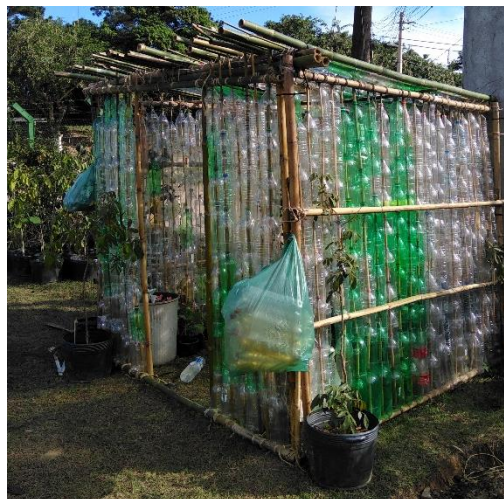
Figure 41: Finished Greenhouse made out of more than 1000 PET bottles, (own archive)
