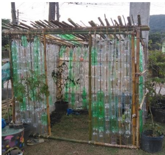
Figure 41: Finished Greenhouse made out of more than 1000 PET bottles, (own archive)
