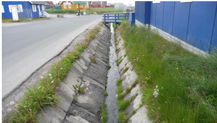
Figure 19: An example of a side ditch. In this case the side ditch is a triangular profile. (RoadEx Network, 2017).
