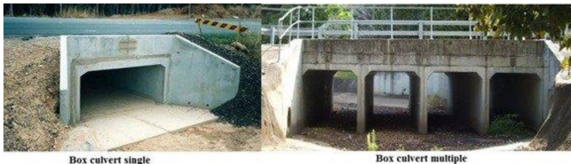
Figure 22: Example of a box culvert. To the right is a single box culvert and to the left is a multiple-box culvert. (The Constructor, 2017).
