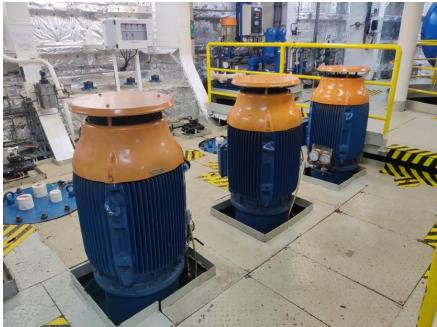
Figure 27 Thruster Room 2 HT LT pump 2 (Starboard side pontoon) Source L.J.M. Verboven (2022)
