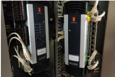
Figure 7 RCU502 and RMP420 installed in Field station (L.J.M. Verboven, 2022).
