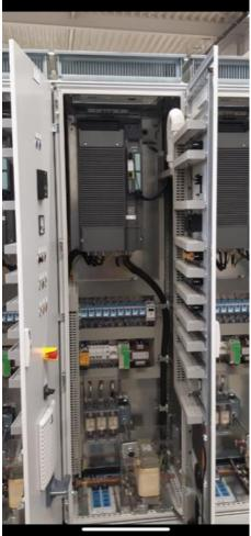
Figure 30 VFD cabinet with one VFD installed inside cabinet including additional parts (OOS International, 2021)
