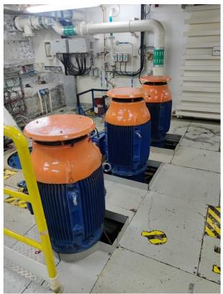
*Figure 26 Thruster Room 1 LT HT pump 3 (Starboard side pontoon). Source L.J.M. Verboven (2022)*
