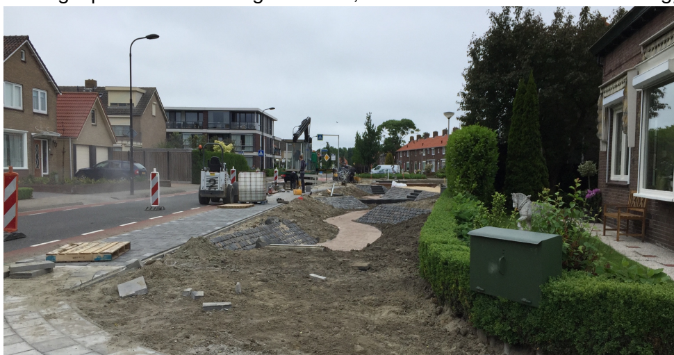
Figure 9 The wadi is currently under construction (May 2017) (picture taken during location visit)
