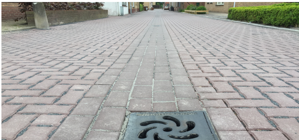
Figure 10 Permeable hardening in the Kerkhoekstraat (picture taken during location visit)
