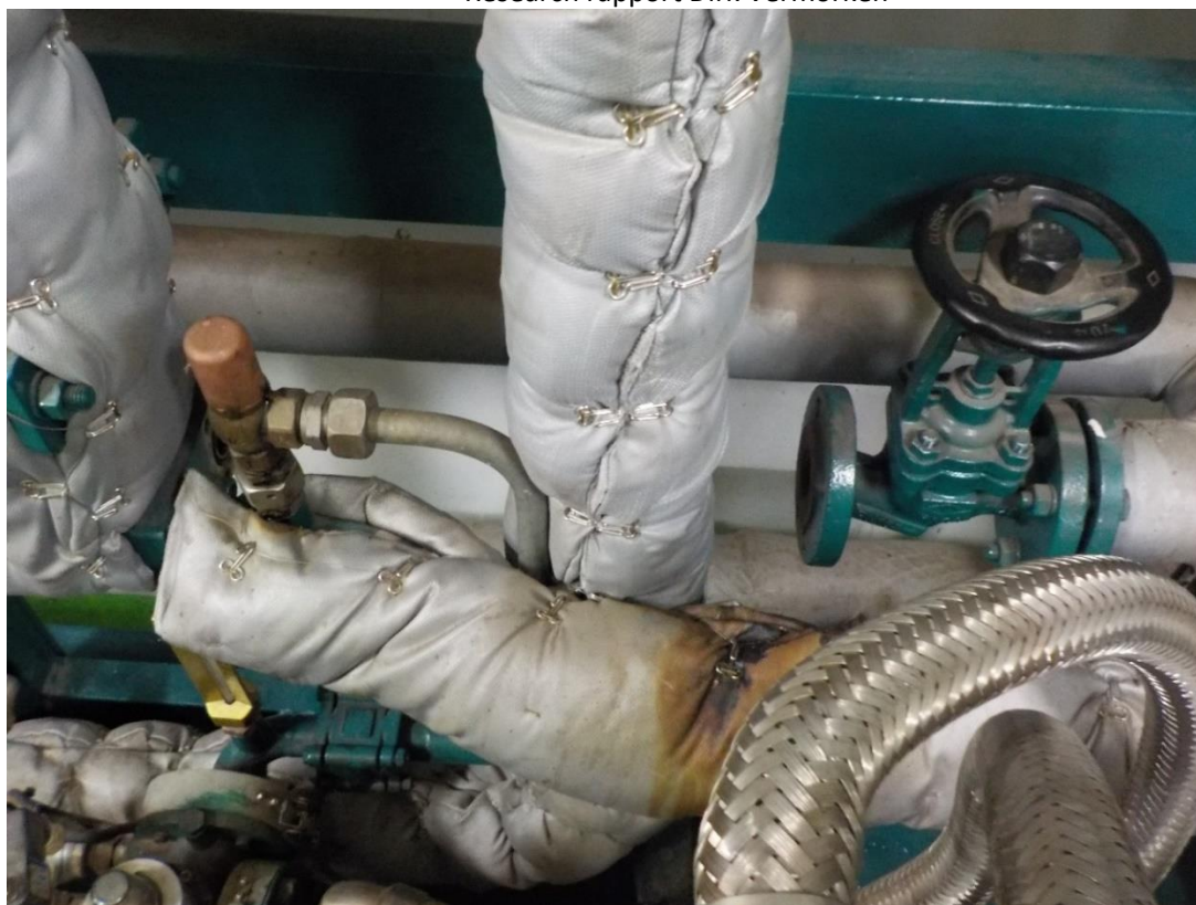
Figure 34 Hot water valve for HFO heat exchanger
