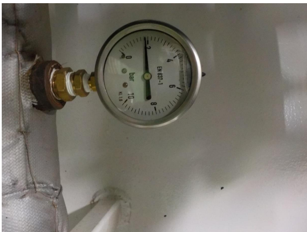
Figure 31 Outlet pressure hot water
