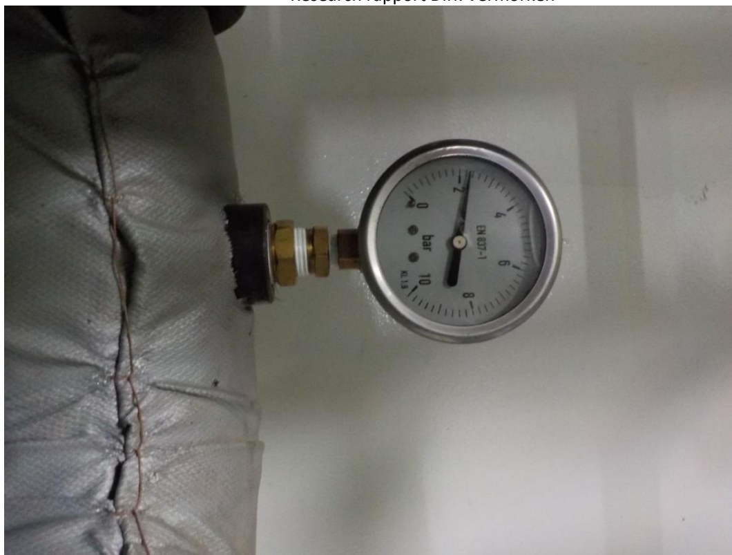
Figure 30 Inlet pressure hot water
