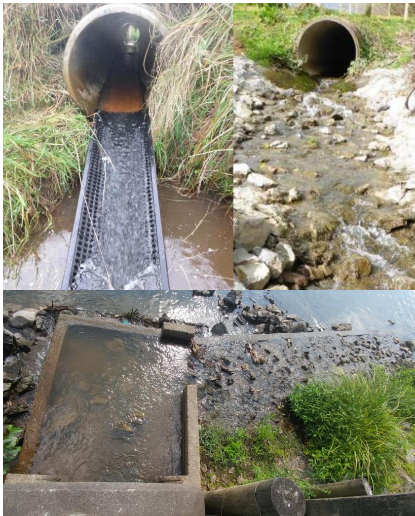
Figure 13: Examples of an artificial substrate ramp (top left), a grouted rock-ramp (top right) and a formal structural design (bottom) (Franklin et al., 2018).
