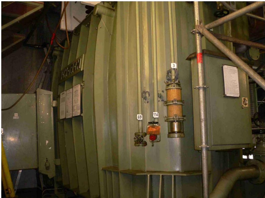
Figure 2-2: Transformer buckling after short circuit (source RWE[10])
